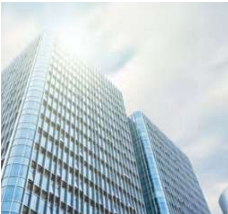
ECSA brings identification of engineering work roadshow to North West
